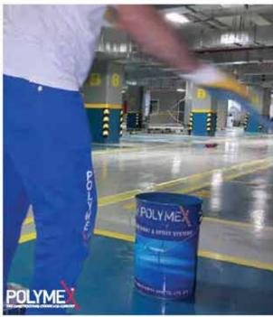
It is used as a primer under any kind of Epoxy – based product. It is a solvent – free, epoxy based, two – component Epoxy primer material.
