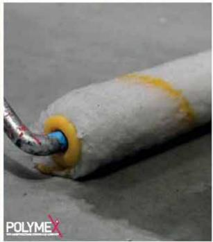
It is a two – component, low viscosity, Solvent Acrylic Resin – based recycling primer. Recycling primer.
