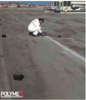
It is an Acrylic Copolymer resin and water – based, single component, ready to use, flexible, white – grey – cream colored, liquid membrane water insulation product which can be easily applied on the floor in any form and painted.
