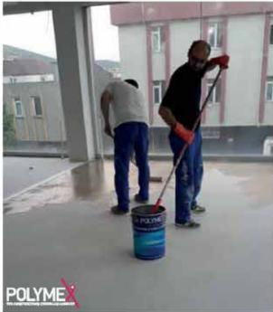
It is an acrylic resin - based, single component, solvent -based acrylic resin primer.
