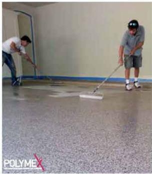
Non -skid floor coating is a dual component, solvent - free, colored, transparent polyurethane based floor coating with a feature lowering humidity. It is a polyurethane non - skid floor coating with high adhesion resistance in comparison with standard floors used by mixing with silica sand and aggregates in different microns.
