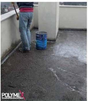
Polyurethane waterproofing membrane is a dual – component, flexible polyurethane insulation membrane which is applied in liquid form for long – term water insulation, having high resistance, and which can be applied and used in cold conditions. It shows the reactionary protective effect together with contact with floor and double mix.
