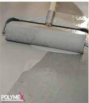
It is a Polyurethane/ Acrylic - Aliphatic based, two component, topcoat Aliphatic paint. Polyurethane topcoat Aliphatic paint.
