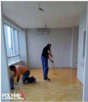
It is a water – based, two - component, solvent free, epoxy based, non-toxic, odorless water-based, protective floor and wall coating paint resistant to saits, oils and some chemicals
