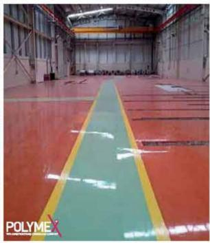
It is a three -component, epoxy based, bright floor covering material.
