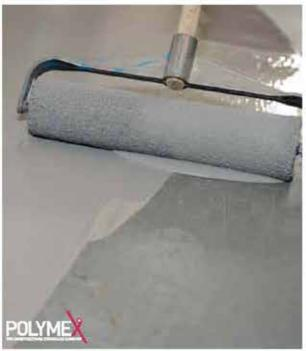
It is an Acrylic copolymer, resin – based, single component, ready to use, flexible, easily applied to any kind of floor, white – grey – cream colored, water insulation material of which surface can be painted. It is compatible with the identification "FIRE RETARDANT COATINGS".
