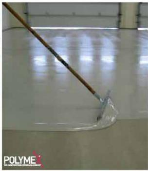
It is a two - component, solvent - free, resin based, PRC floor coating material.
